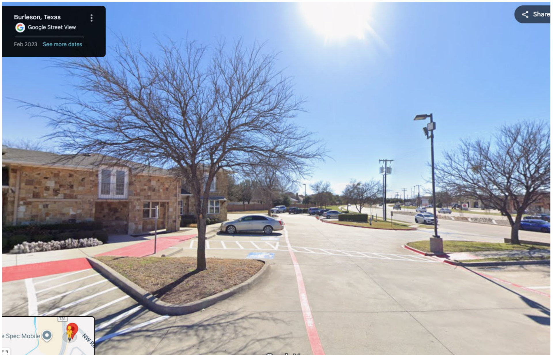
Looking south from the parking lot near the current entrance toward where the portable building would be located
